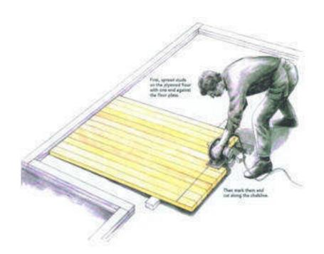
Batch-cutting' is even more efficient if you use a portable 'DIY' electric power-saw rather than a hand-saw; especially as 'batch-cutting' minimizes the time when electric power is needed onsite if a generator has to be used! It is very rare for the cutting of framing and sheathing to extend beyond a day's work for anything less than a 250 m² house when properly planned and executed!
