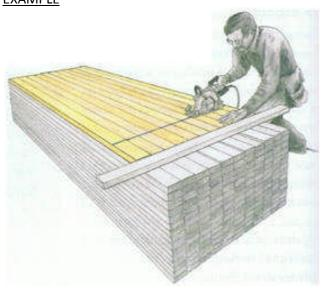
Whilst it should be obvious to one-and-all that it is quicker to cut two lengths of timber at once than it is to measure and cut each length separately  $\sim$  it is <u>very</u> much quicker to cut batches of 15 - 20 pieces to length each time by using a simple 'jig'!
